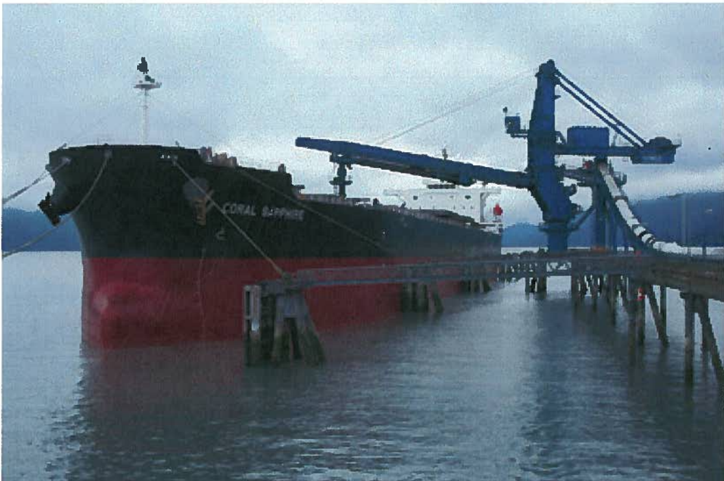
Figure 3: Conveyor system and transport vessel in Resurrection Bay.
