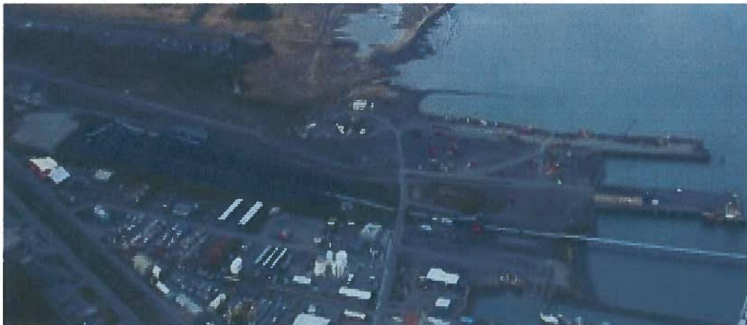
Figure 1: The two coal stockpiles (left portion of this photo) and conveyor system extending into Resurrection Bay (right portion of this photo).
