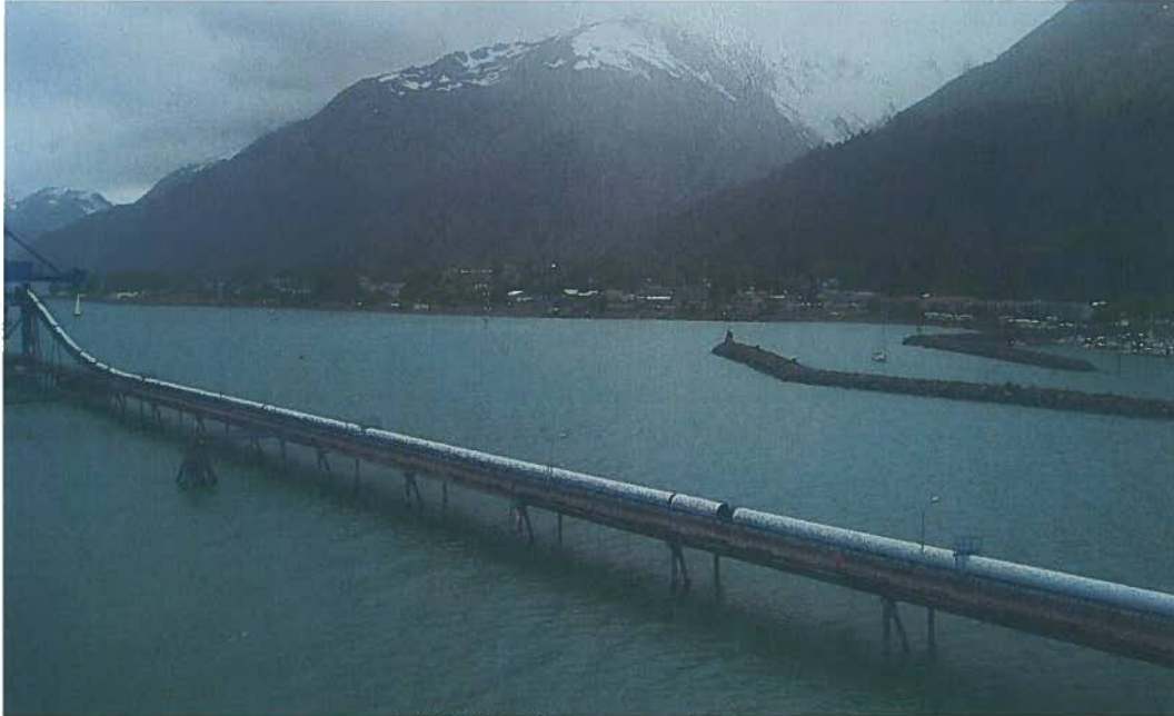
Figure 2: Conveyor system extending over Resurrection Bay.
